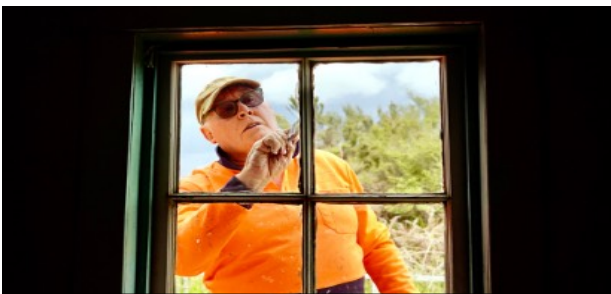
Oliver Young concentrating on painting a window in Gill's Cottage
