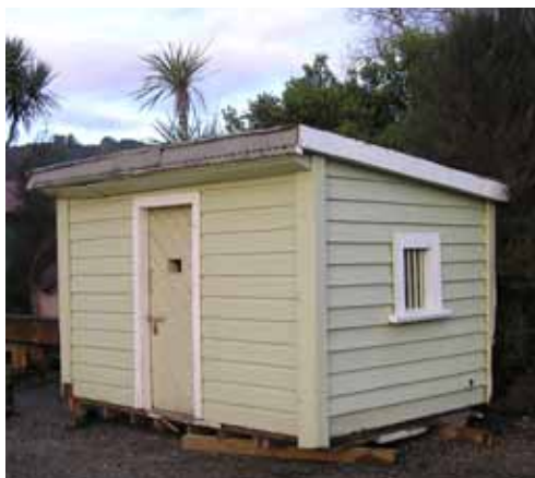
The lock-up sitting in the DOC compound at Reefton, awaiting some attention and a likely return to the Waiuta.
